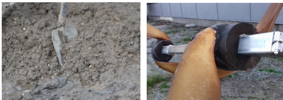
Figure 1: a) Sand and gravel removed from digester and b) damaged stirrer
