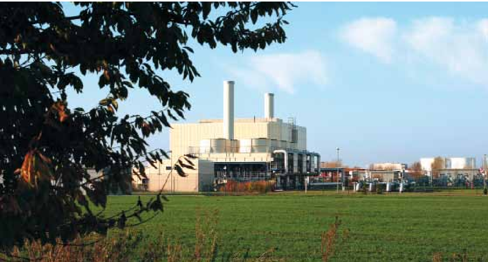
Transmission plant of the underground gas storage of VNG AG in Bad Lauchstedt/Saxony-Anhalt, photo: VNG AG
