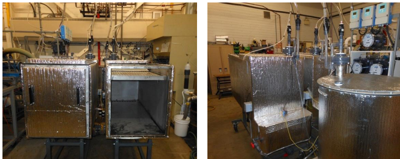
Figure 8.7-1: Dry batch digestion pilot plant at AITF. The pictures show the front of the system (left) and back (right) with a round percolate digester in the back (Source: InnoTech)
